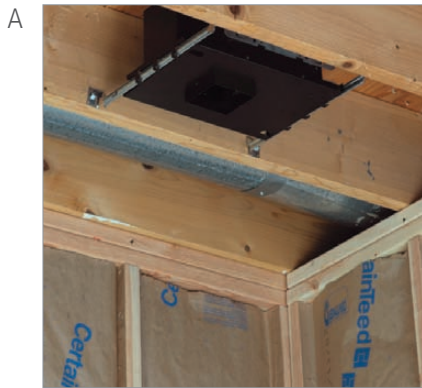
Install housing to the ceiling joists with the adjustable steel hanger bars (shown above).
