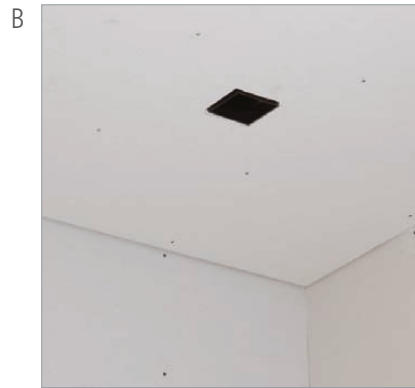
Mount gypsum board to ceiling and walls.
